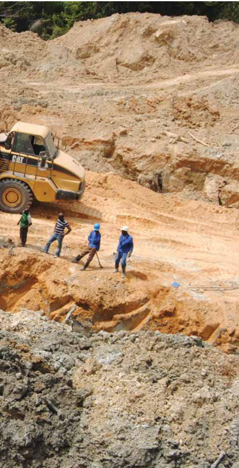
Waste stripping in progress at Kundu Central Dyke.
